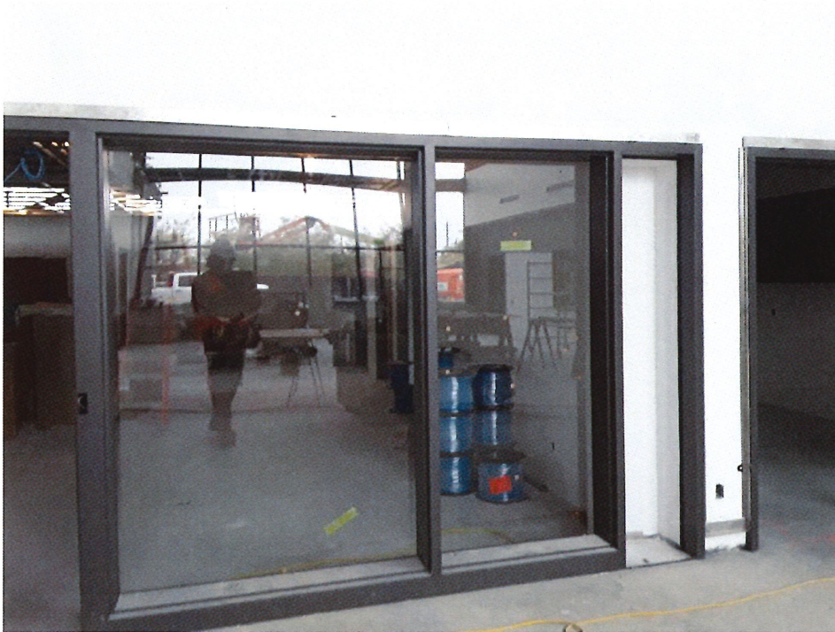
Glazing installation complete at hollow metal frame areas
