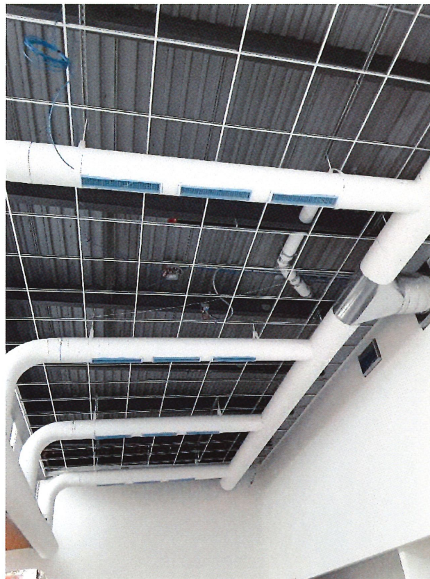
Community Meeting Room - exposed ductwork painted with louvre installation
