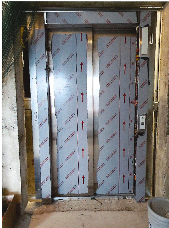
Ground Floor Elevator - Door & frame installations
