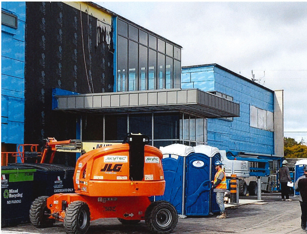
East Elevation (looking north) – Installation of zinc cladding at staff entry canopy
