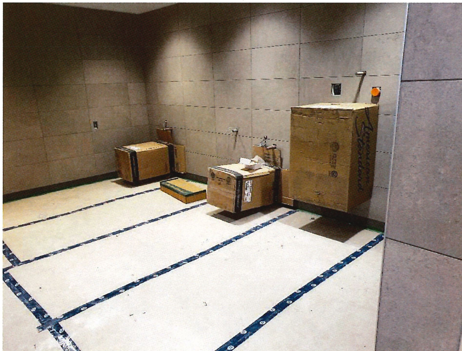
Male Locker Rm – Completed tile & plumbing fixture installations (boxed for protection)
