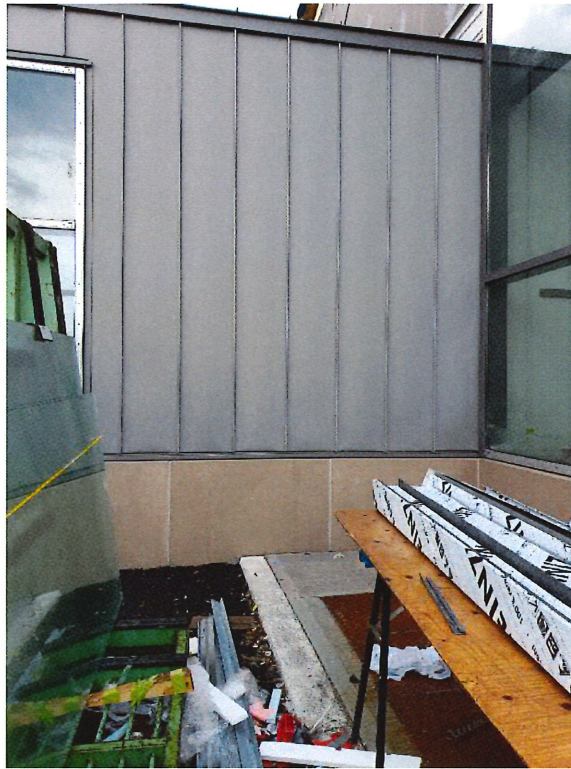
South Elevation (at staff entry vestibule) – Installation of zinc cladding
