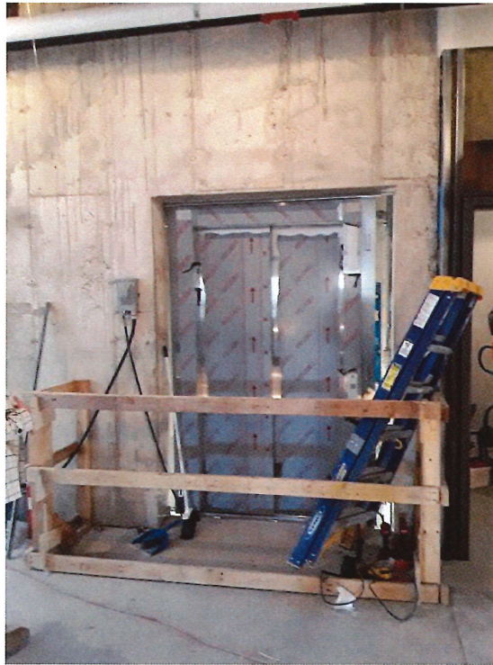
2 nd Floor Elevator - Door & frame installations
