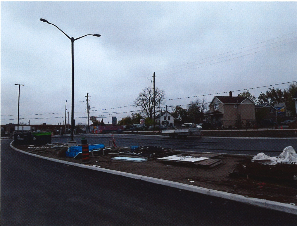
East Elevation (looking east) – Parking light standard installations
